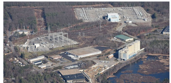
Substation in Ayer, Mass.
